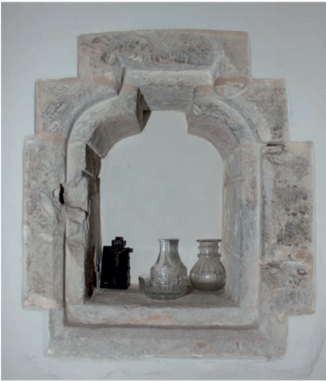
22 - Above, the Ambry in the south wall. Vestiges of medieval paint and plaster remain associated with this furnishing.
