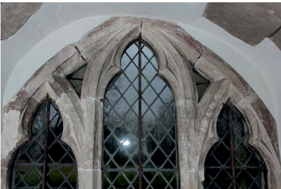
7 - Left, the upper part of the east window. Traces of medieval paint (red) are especially apparent toward the top of the window tracery. There are a number of open joints in the tracery, indicating structural movement.
